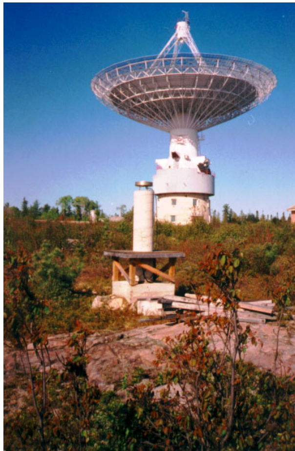
Figure 2. Algonquin Antenna with co-located GPS Antenna
