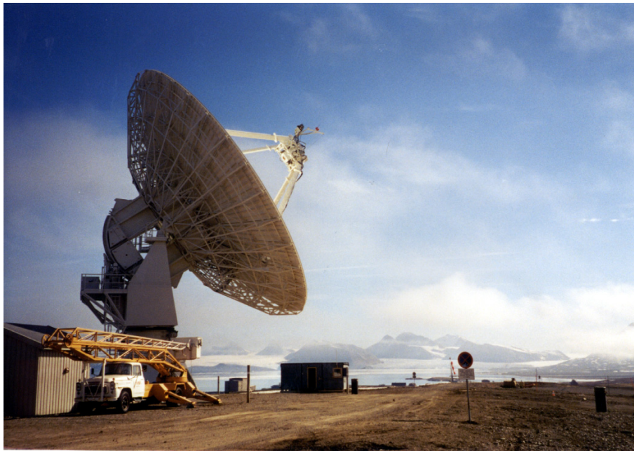
Figure 1. The VLBI antenna at Ny-Ålesund. View is approximately from south-west to north-east. The 20-m radio telescope is located on a small plateau approximately 1.5 km west of the village of Ny-Ålesund at about 45 m above sea level. The small green house seen in the middle of the picture is the control building of the airport, with part of the runway visible in the rightmost corner of the picture. The two black pillars to the right of the airport building and in the right lower corner are well-isolated pillars of the local control network. Photo taken in July 1998.
