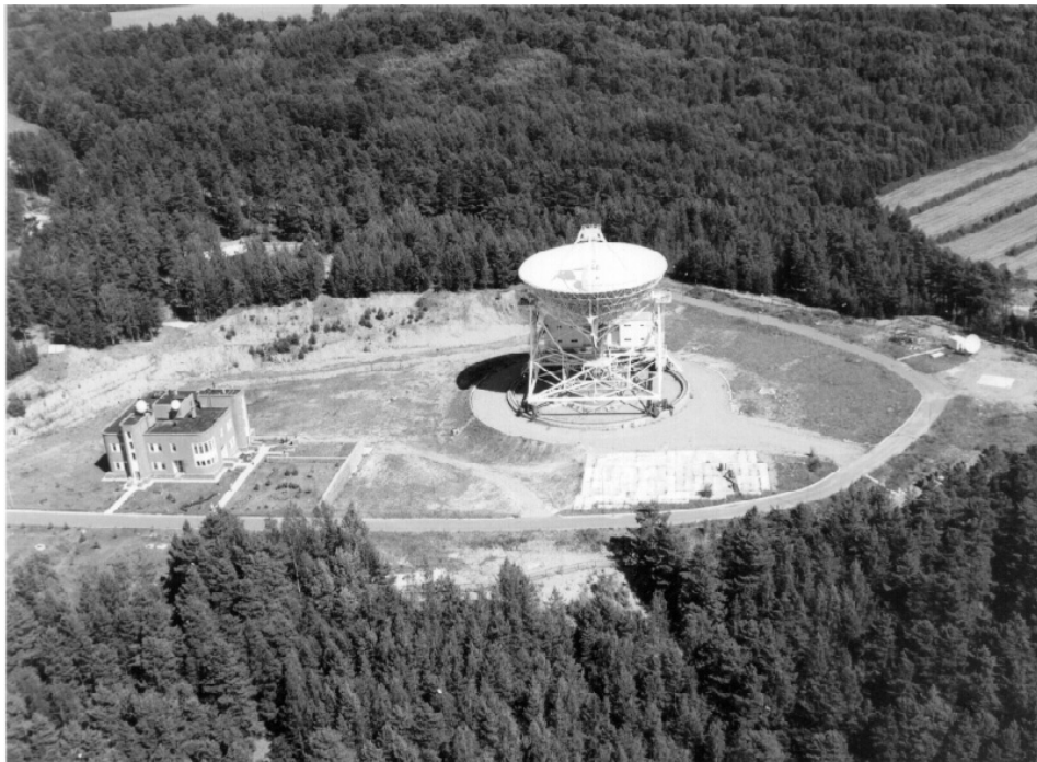
Figure 2. Svetloe station: laboratory building and radiotelescope RTF-32.
