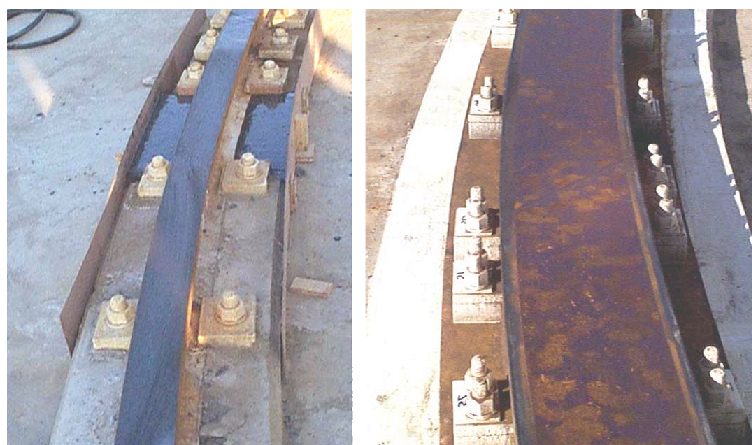
Figure 3. Azimuth rail replacement (Left: before Right: current).
