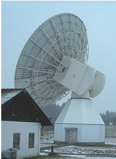
Figure 1. 20m radiotelescope with new insulation of the concrete supporting construction.
