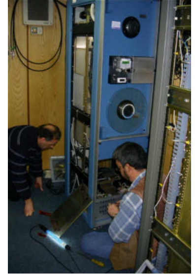
Figure 3. Installation of the thin tape equipment
