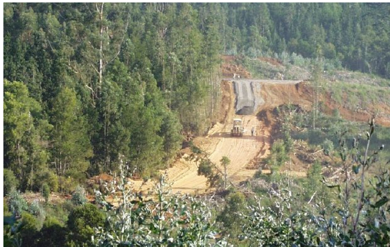
Figure 1. March 23, 2001. The access road to the TIGO platform is being prepared.
