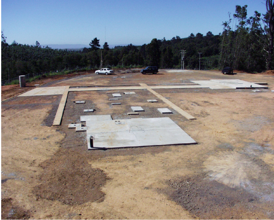
Figure 3. December 3, 2001. The platform is prepared with foundations, underground cable ducts and monuments for the reception of the TIGO containers with their telescopes and instruments.
