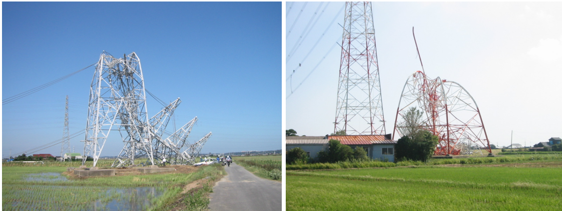
Figure 1. High voltage electric power transmission towers were pulled down by strong wind of the typhoon. Photo were taken by R. Ichikawa at Itako.
