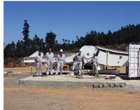
Figure 4. February 4, 2002. The radiotelescope is being installed. The 18-ton main part of the radiotelescope had been moved only with muscle power. The reference marker of the VLBI monument is now occupied by the radiotelescope static part.
