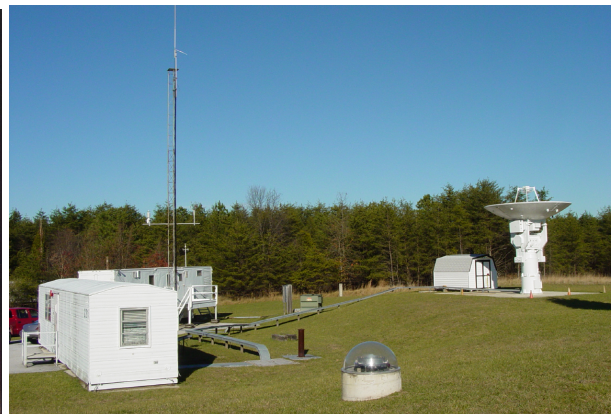
Figure 2. New permanent MV-3 antenna.
