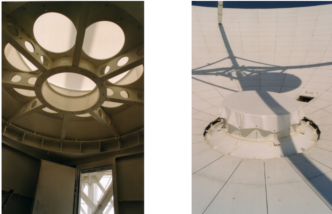
Figure 1 – Left : View of the cover of the vertex room. Eight receivers can be permanently mounted, one for each of the external holes. The hole on-axis will host receivers under test. Right : View of the top of the vertex room.
