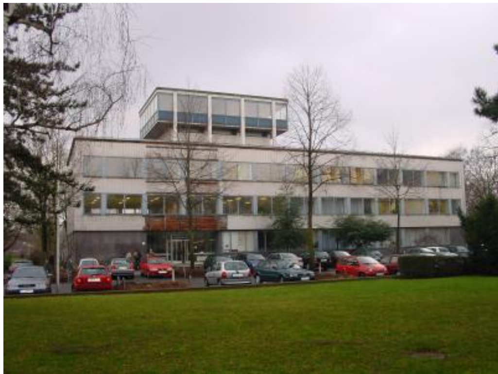
Figure 1. Building of the Geodetic Institute
