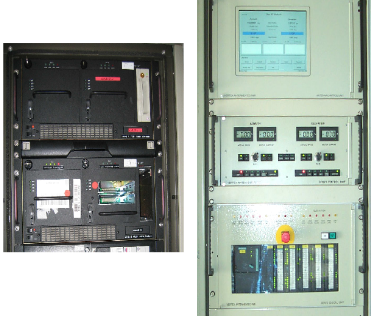
Figure 1. 2 MK5A systems, one with modifications for the Intensives (left); New Antenna Control Unit (ACU) (right)
