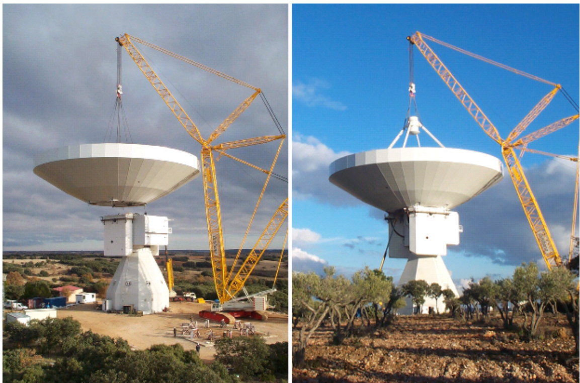
Figure 1. Erection of the new 40 meter radiotelescope of OAN at Yebes (Guadalajara, Spain).
