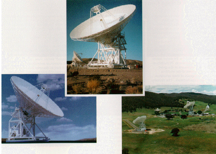
Figure 1. This figure shows the three high-efficiency antennas in the subnet: Goldstone is in the center; Robledo, Spain is in the lower left; and Tidbinbilla, Australia is on the lower right. These antennas were designed to have an optimum efficiency at X-band (8.4 GHz), which was to become the standard downlink frequency for solar-system exploration. An important secondary objective was to have a reasonable efficiency at Ka-band (32 GHz) thereby allowing for possible future use at the next highest band allocated for deep space communications. The subnet was completed in 1986 in time for the Voyager encounter with Uranus.
