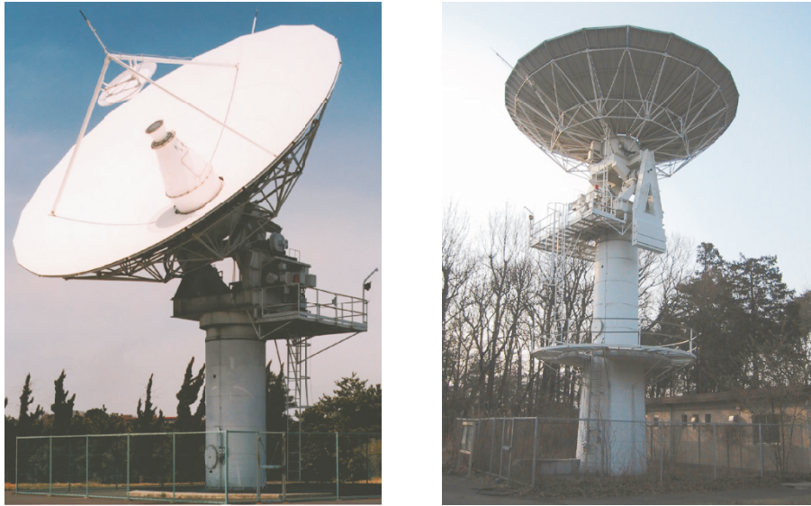
Figure 2. 11-m VLBI antennas at Kashima (left) and Koganei (right).
