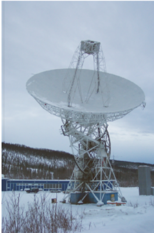
Figure 1. Gilmore Creek Geophysical Observatory's telescope and building, Fairbanks, Alaska.
