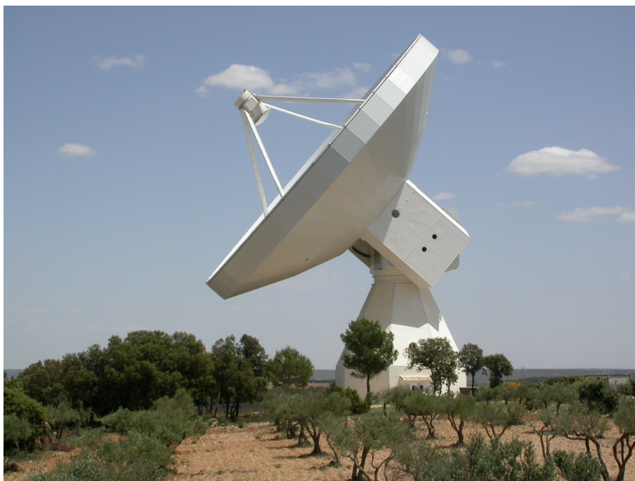
Figure 1. The new 40-m radiotelescope of OAN at Yebes, for geodetic and astronomical VLBI.
