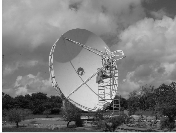
Figure 1. Fortaleza's station team repairing the 14.2 m antenna
