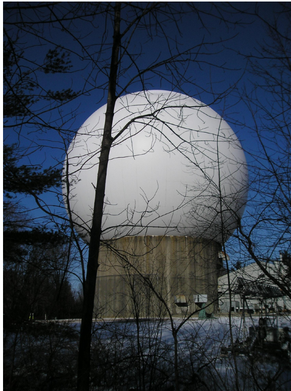
Figure 1. The radome of the Westford antenna.
