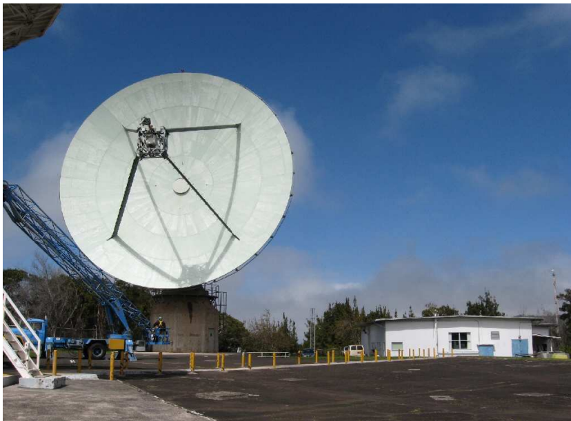
Figure 1. KPGO 20m antenna and operations building.
