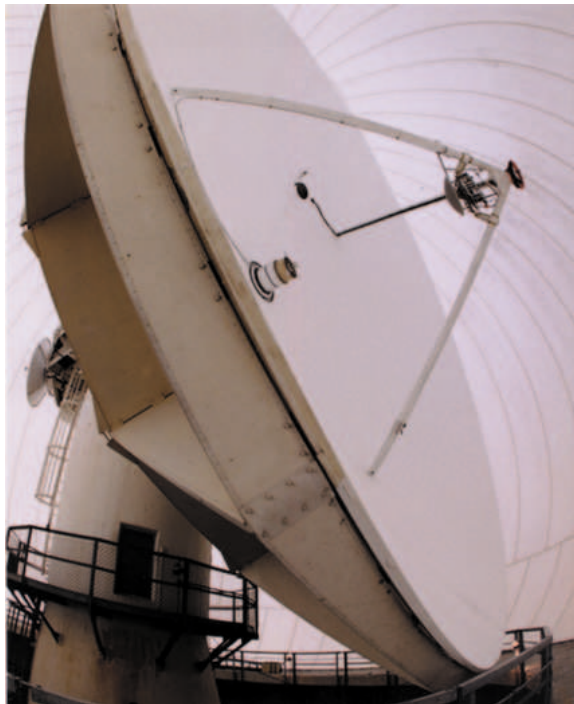
Figure 2. Wide-angle view of Westford antenna inside the radome. The VLBI S/X receiver is located at the prime focus. The subreflector in front of the receiver is installed when observing with the TAL receiver (see Section 4), which is located at the Cassegrain focus.
