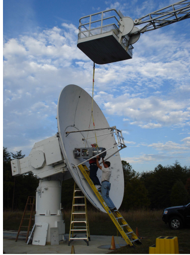
Figure 1. Jay Redmond and Bruce Whittier installing the Dewar on the 5 m MV-3 antenna.
