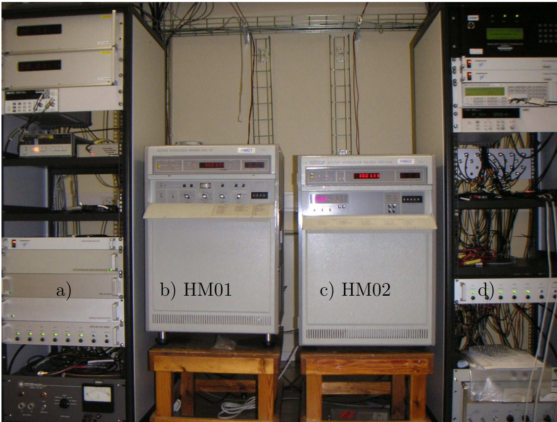
Figure 2. Time lab at Onsala: a) Rack with, for example, GPS TAC, several 5 MHz distributions, pulse distribution unit, b) HM01: Kvarz CHI-75 installed in March 1997, c) HM02 Kvarz CHI-75A installed in April 2007, d) Rack with, for example, GPS time receivers, AOG (Auxilliary Output Generator) for UTC generation, and space for the Cesium clock (to be installed during 2008).
