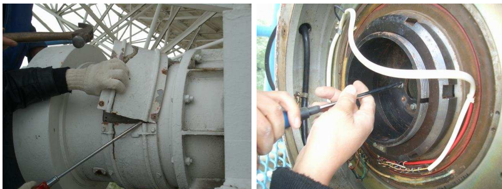
Figure 2. Fastening the elevation encoder screw in December 2008.
