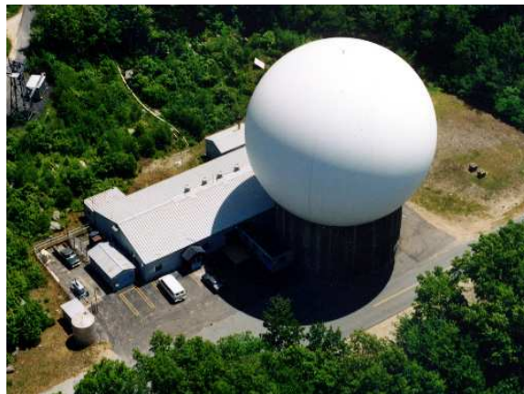
Figure 1. The radome of the Westford antenna.
