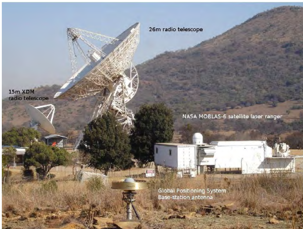
Figure 1. HartRAO fiducial site: space geodetic techniques of VLBI, GNSS, and SLR. (Credit: M. Gaylard)
