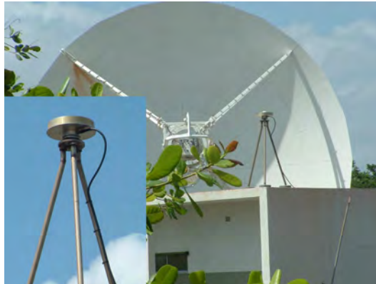
Figure 3. Detail of GPS antenna placed over the main building.
