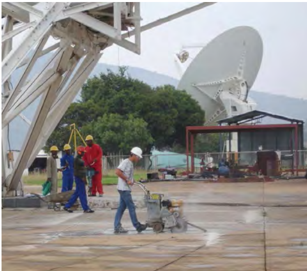
Figure 4. Groundbreaking: cutting the slab for the construction of the 26-m's A-frame support; in the background, the XDM is being put through its paces using the adapted 26-m observing scheduler. (Credit: M. Gaylard)
