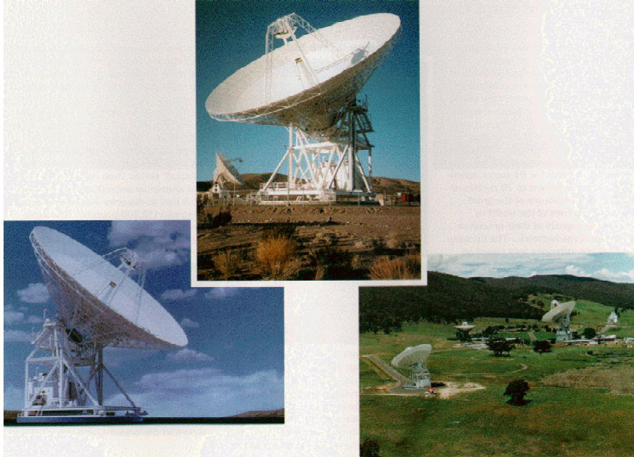
Figure 1. This figure shows the three high-efficiency antennas in the subnet: Goldstone is in the center; Robledo, Spain is on the lower left; and Tidbinbilla, Australia is on the lower right. These antennas were designed to have an optimum efficiency at X-band (8.4 GHz), which was to become the standard downlink frequency for solar-system exploration. An important secondary objective was to have a reasonable efficiency at Ka-band (32 GHz) thereby allowing for possible future use at the next highest band allocated for deep space communications. The subnet was completed in 1986 in time for the Voyager encounter with Uranus.
