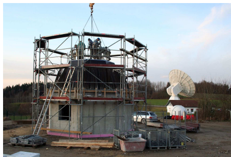
Figure 2. Construction of the concrete tower for the TWIN telescopes
