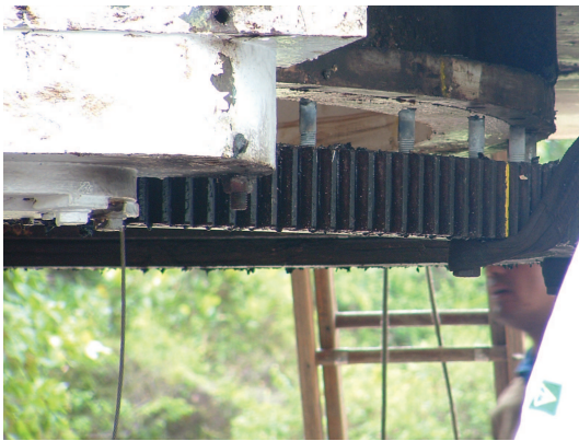
Figure 3. Old bearing being removed.
