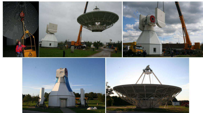
Figure 1. Repair of the bearings of the 20-m radio telescope.
