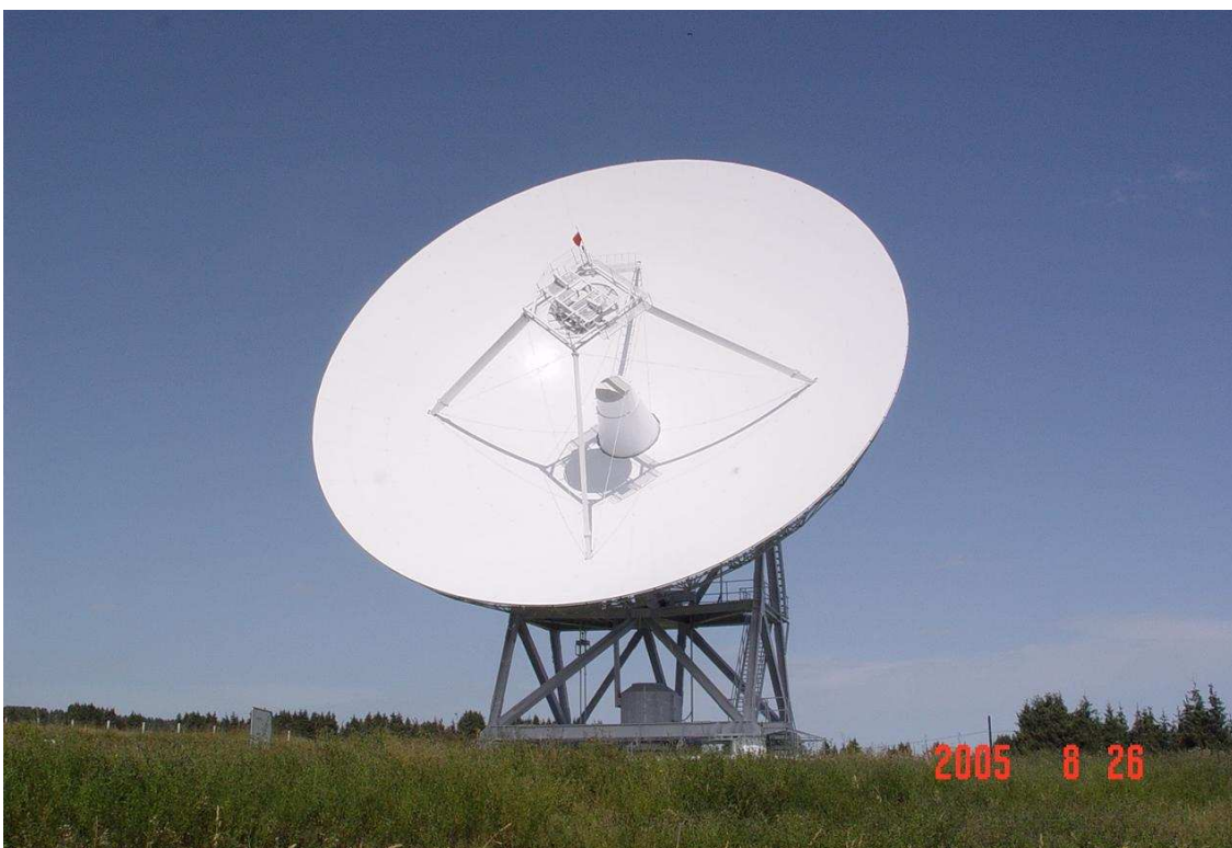
Figure 2. The 25-m, modified Cassegrain radio telescope of the Xinjiang Astronomical Observatory.
