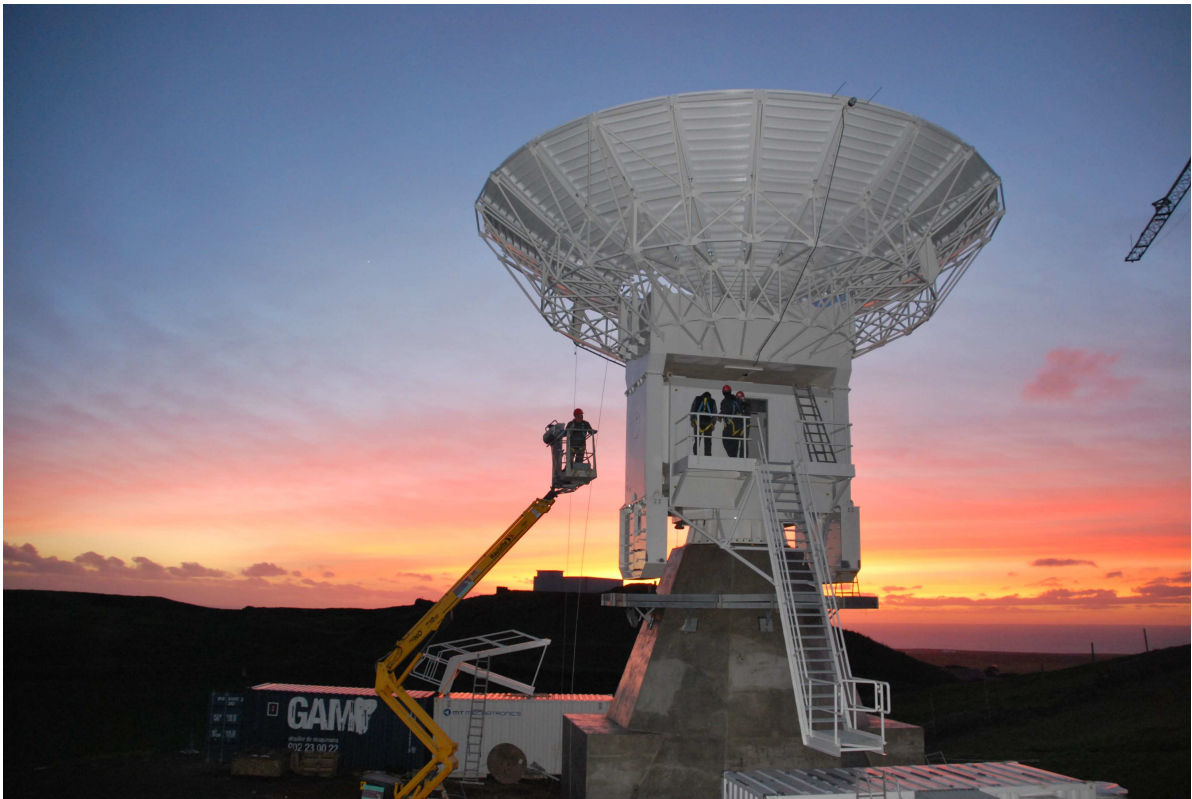
Fig. 3 Status of construction of the RAEGE antenna in Santa Maria (Azores islands, Portugal).
