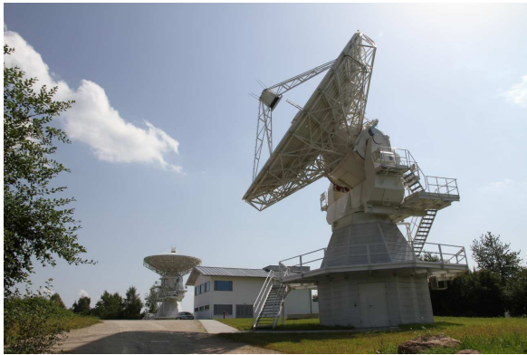
Fig. 2 The Twin radio Telescope Wettzell (TTW) as Wettzell's realization of a complete VLBI2010 conformity.
