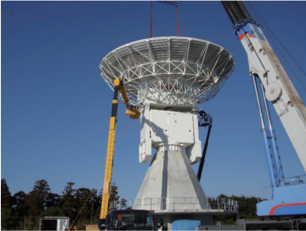
Fig. 5 Construction of the antenna.
