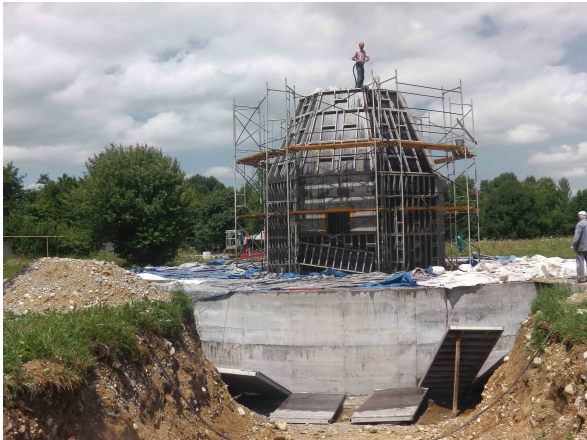
Fig. 4 Autumn 2013, building in progress.
