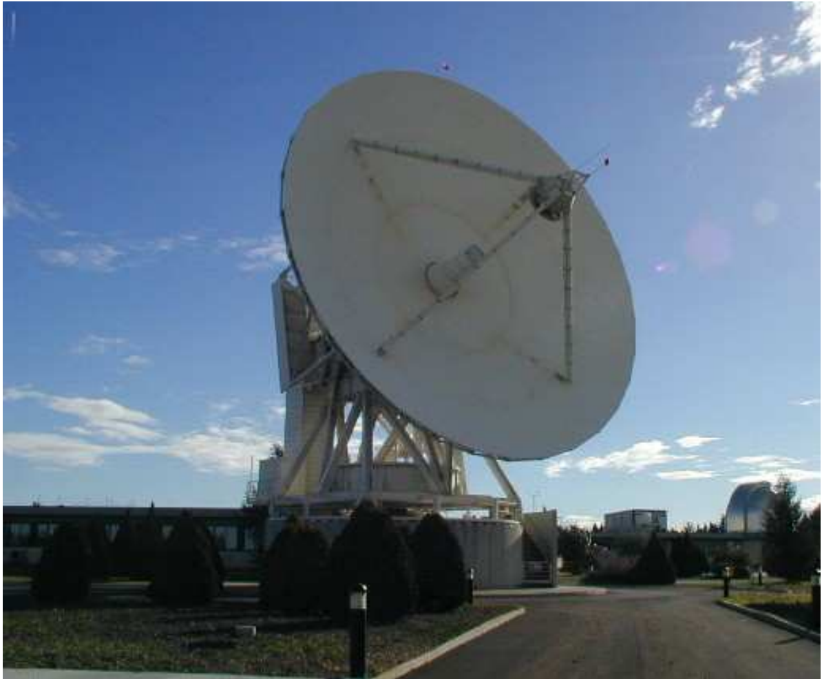
Fig. 1 VLBI antenna and MLRO dome.
