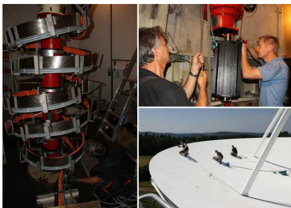
Fig. 1 Some replacement work at the RTW: new setup of the cable wrap (left), replacement of the gears and motors (upper right), and new varnishing of the reflector surface (lower right).
