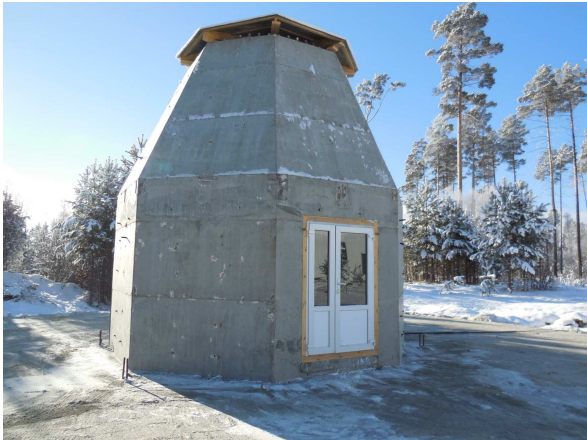
Fig. 5 Antenna tower for 13.2-m dish.
