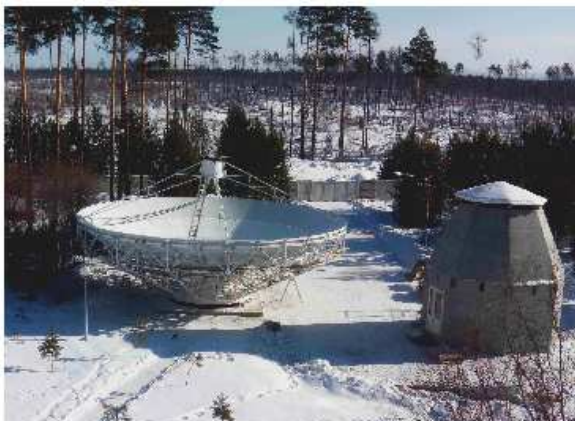
Fig. 6 Main reflector 13.2-m and antenna tower.
