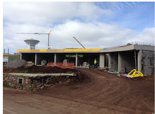
Fig. 4 Status of construction of the control and auxiliary buildings of the RAEGE station in Santa Maria.
