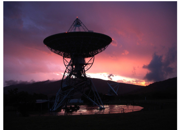
Fig. 1 The HartRAO 26 m under repair after a thunderstorm and lightning strike during the Ultra-rapid R1579 on 2 April 2013 (with the 15 m in the background).
