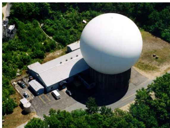
Fig. 1 The radome of the Westford antenna.
