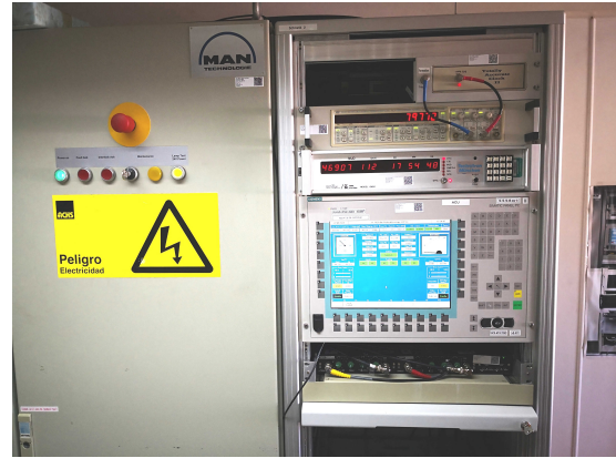
Fig. 5 Servo cabinet with antenna control unit inside the AGGO-2 VLBI operation container.
