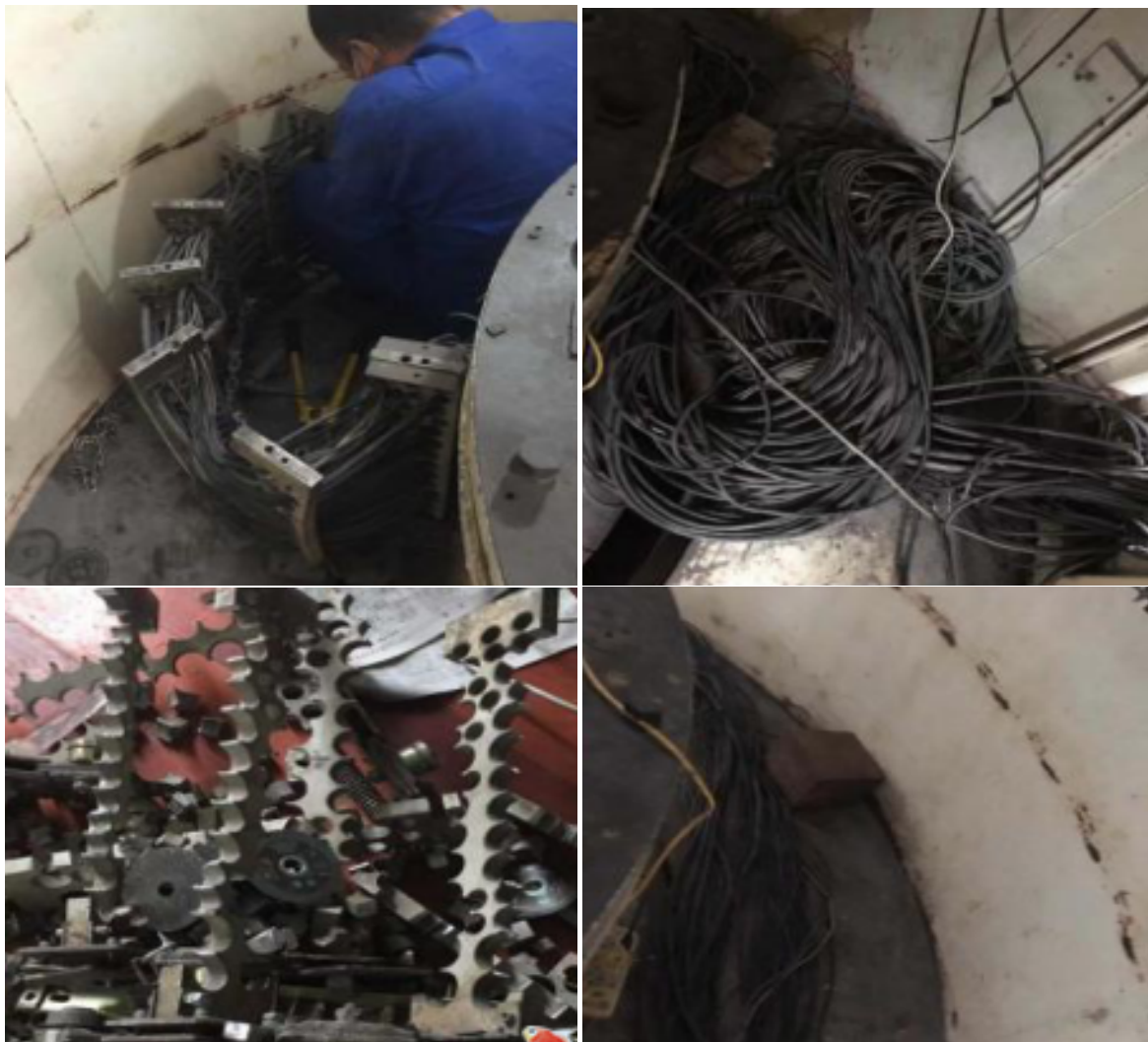
Fig. 1 The antenna chain removal, completed.
