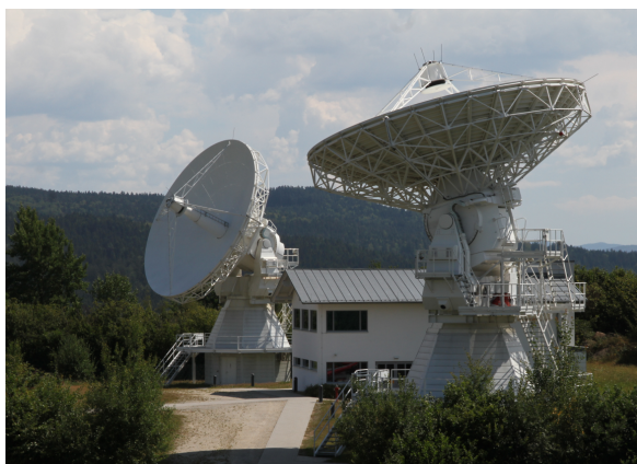
Fig. 4 The Wettzell Twin Telescope with its two 13.2-m antennas (Wn in the front) and the control building.
