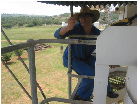
Fig. 5 Jacques Grobler greasing the 15-m antenna's gears.
