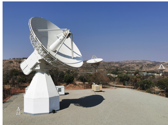
Fig. 1 The HartRAO trio (from left to right): the VGOS, 26-m, and 15-m antennas. The newly installed VGOS backup generator is visible next to the shadow of the VGOS antenna.
