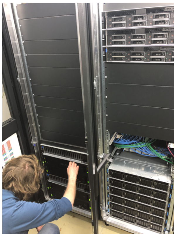
Fig. 2 Installation of the new correlation facility at Wettzell observatory.
