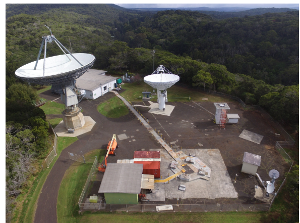
Fig. 2 KPGO site overview.
