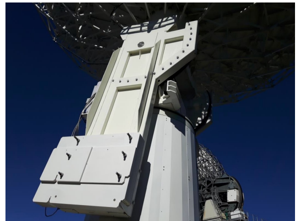
Fig. 5 12-m telescope counterweight rebalance effort.
