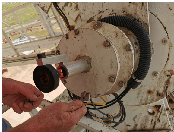
Fig. 7 Site tie: multi-prism pillar being installed co-axially on the 26-m telescope’s shaft.
