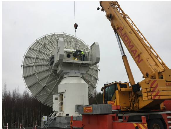
Fig. 2 Receiver installation on the VGOS radio telescope. Photo: Nataliya Zubko
