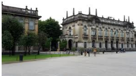
Fig. 1 Politecnico di Milano Building 3, where the AC PMD is hosted.
