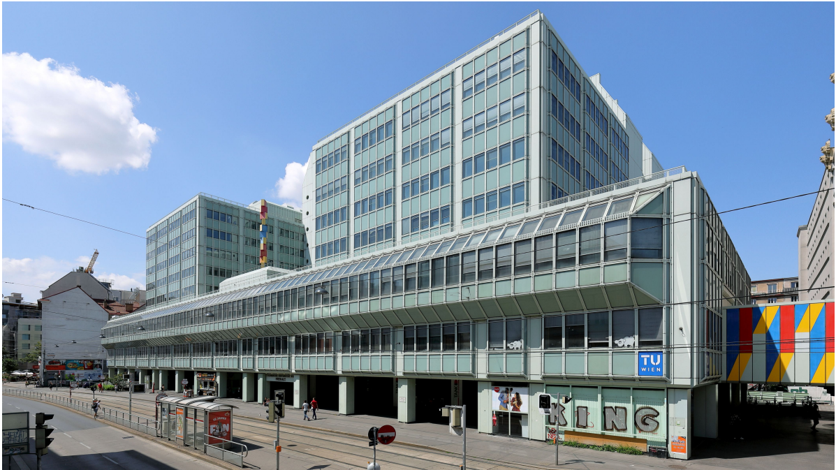
Fig. 1 The “Freihaus” of TU Wien (second floor, yellow area) is the new home of the research unit Higher Geodesy of the Department of Geodesy and Geoinformation since September 2019.
