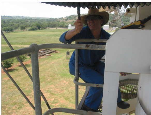
Fig. 5 Jacques Grobler greasing the 15-m antenna's gears.
