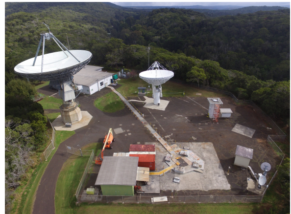
Fig. 2 KPGO site overview.
