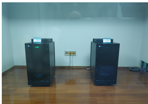
Fig. 6 The new hydrogen clock room.
