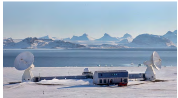
Fig. 2 The geodetic observatory's Brandal site with 13-m twin telescopes. From left to right: Ny-Ålesund 13-m North antenna (Nn), SLR dome, operations building, and Ny-Ålesund 13-m South antenna (Ns). (Image: Bjorn-Owe Holmberg)
