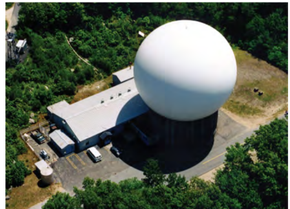
Fig. 1 Aerial view of the radome and facilities of the Westford antenna at MIT Haystack Observatory. (For scale, the diameter of the radome, which veils the 18.3-m diameter antenna, is 28 m.)
