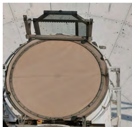
Fig. 4 A brand new cover for the 26-m antenna's feedcone.
