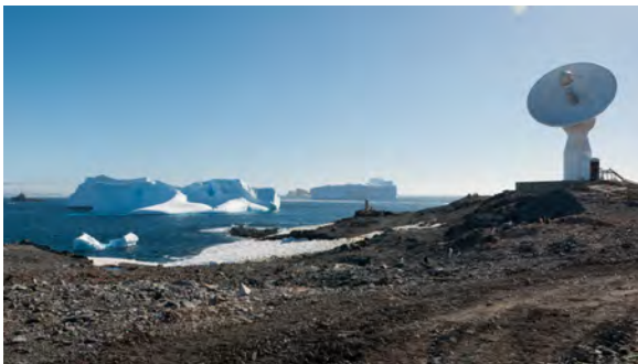
Fig. 2 The nine-meter VLBI antenna of O'Higgins Antarctic Station. [Credit: DLR (CC BY-NC-ND 3.0)]
