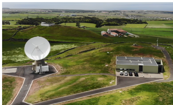
Fig. 1 RAEGE Santa Maria radio telescope and control building.
