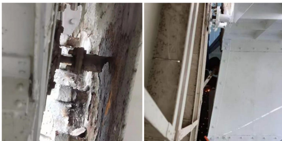
Fig. 2 Replacement of supporting bars.
