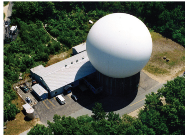
Fig. 1 Aerial view of the radome and facilities of the Westford antenna at MIT Haystack Observatory. (For scale, the diameter of the radome, which veils the 18.3-m diameter antenna, is 28 m.)
