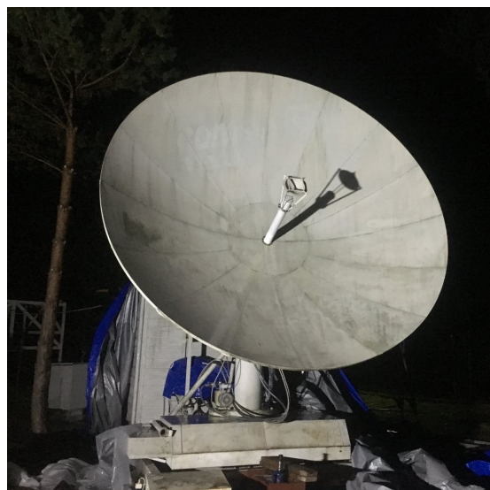
Fig. 1 The TESLA S11 DD 424 ground-based satellite communication station.
