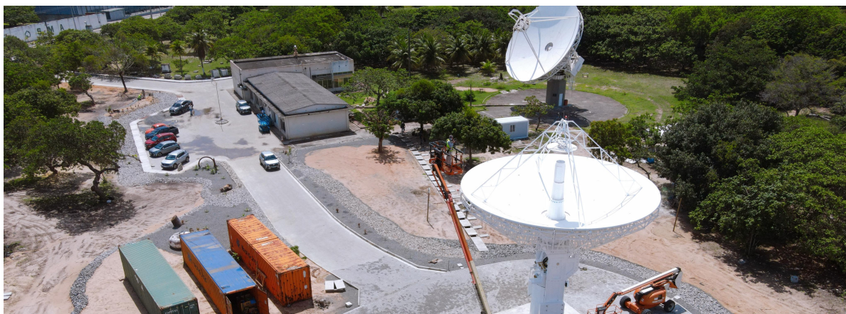
Fig. 2 Overview of the Fortaleza Geodetic Observatory (ROEN/FGO), showing the newly installed 12-meter VGOS antenna (foreground) and the legacy 14.2-meter antenna (background). Photo taken during the final phase of installation, early 2025.
