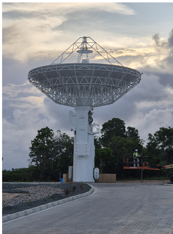
Fig. 1 Installation of the 12-meter VGOS antenna at Fortaleza Geodetic Observatory (FGO/ROEN).
