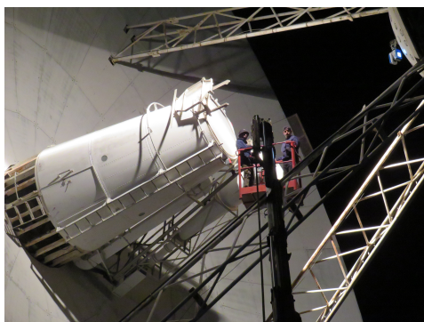
Fig. 6 TLS installation for gravitational deformation survey of the 26-m antenna.
