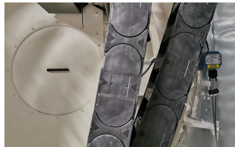
Fig. 8 VGOS pressure sensor installed in the elevation cabin at its reference height.
