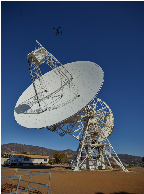
Fig. 4 Ho telescope being surveyed via aerial photogrammetry.
