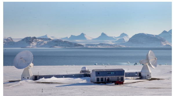
Fig. 1 The geodetic observatory's Brandal site with 13-m twin telescopes. From left to right: Ny-Ålesund 13-m North antenna (Nn), SLR dome, operations building, and Ny-Ålesund 13-m South antenna (Ns). (Image: Bjorn-Owe Holmberg)
