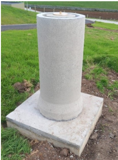
Fig. 6 Local-tie pillar installed at Santa Maria station.
