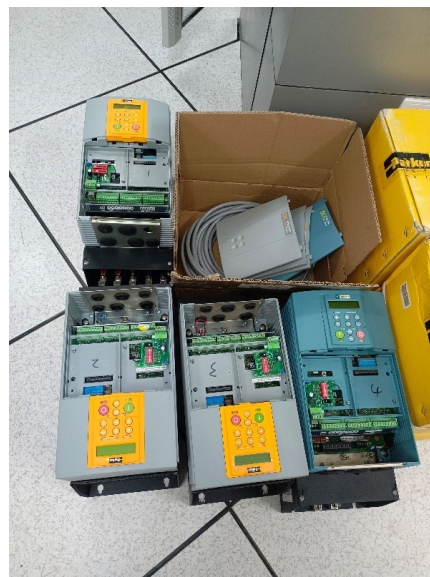
Fig. 1 Images show the removal of the old drive device.
