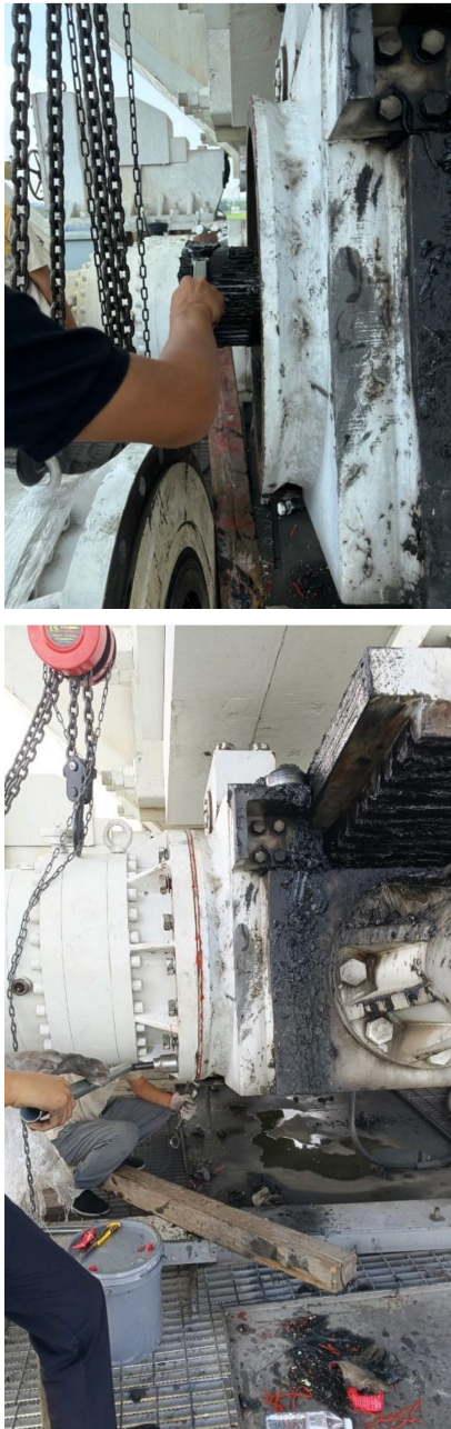
Fig. 3 Repairing the #2 reducer of elevation.
