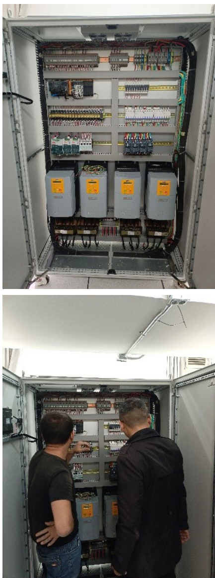
Fig. 2 Images show the installation of the new drive device.
